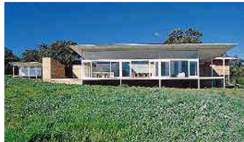
North elevation with guest house at left (Martin Farquharson, Architecture Media Pty Ltd)
