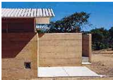
Rammed earth walls in the south-east corner (Martin Farquharson, Architecture Media Pty Ltd)
