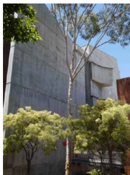
East Elevation (John Stephens 2010)
