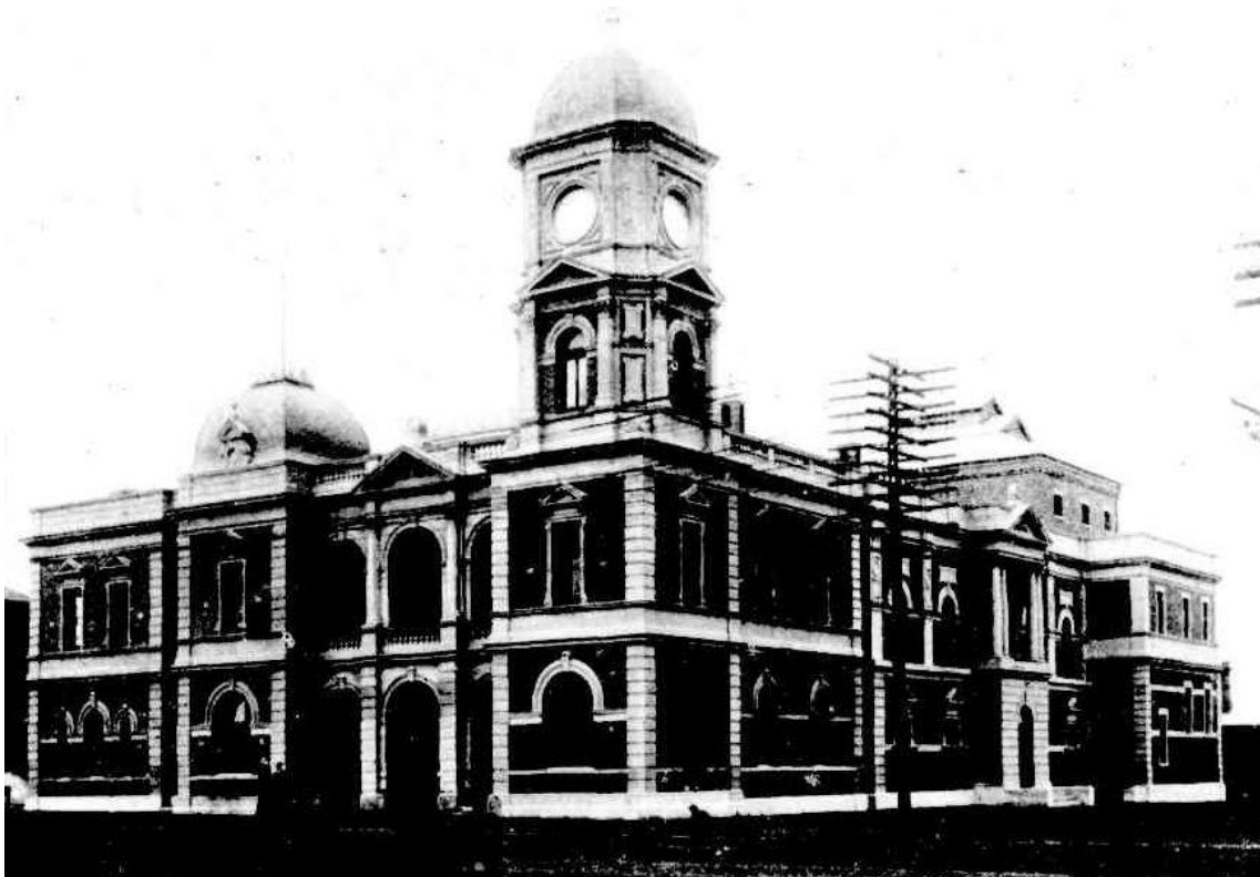
Boulder Town Hall completed in 1908 ( Kalgoorlie Western Argus , 14 July 1908, p.19)
