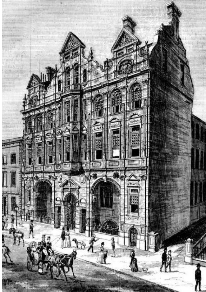
Offices for Stephen, Jaques and Stephen's, O'Connell Street, Sydney – designed by 'rising' architects Coward & Bell ( Australian Town & Country Journal , 8 September 1888, p.31).
