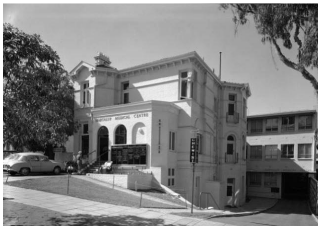
Pictured in a substantially altered form as a medical centre at 254 St George's Terrace in 1959, Salway designed Martalup in 1897 for lawyer-politician George Leake. It has been demolished. (SLWA 113086PD).
