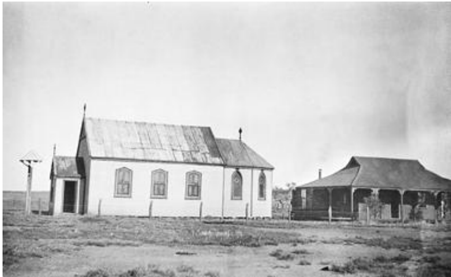
St Saviour Church Yalgoo, at left of photo, opened on 1 September 1907, but has been demolished (courtesy of Dominican Sisters, Doubleview).
