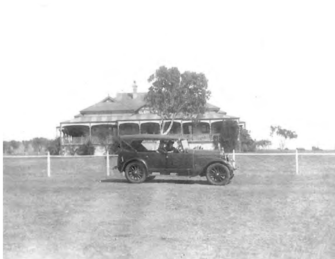
Glengarry homestead built in 1912 for Jack Grant with Shephard's Buick in the foreground, 1927 (courtesy Faye Smart, Conservation Plan for Glengarry Homesteads (1852) & (1912) , John Taylor Architect, 2004, p.41)
