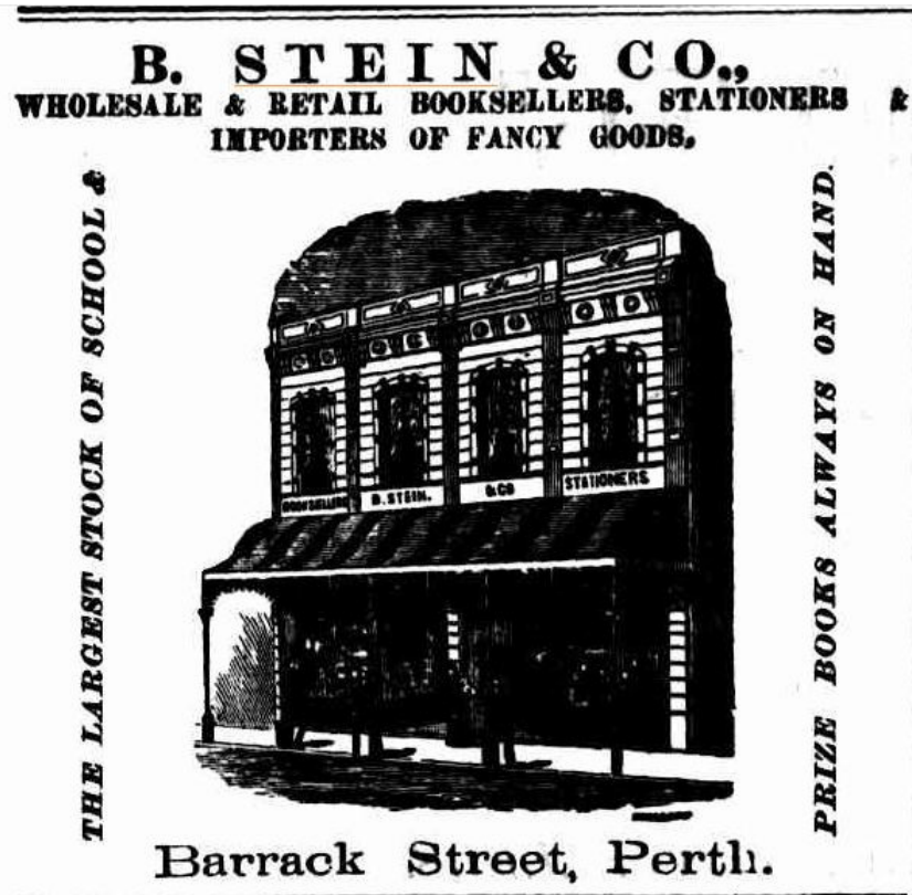
Designed by Harry Trigg, Bernard Stein's Barrack Street, Perth premises were located on the site now occupied by the Bon Marche Arcade (The Western Mail, 18 December 1886, p.13).
