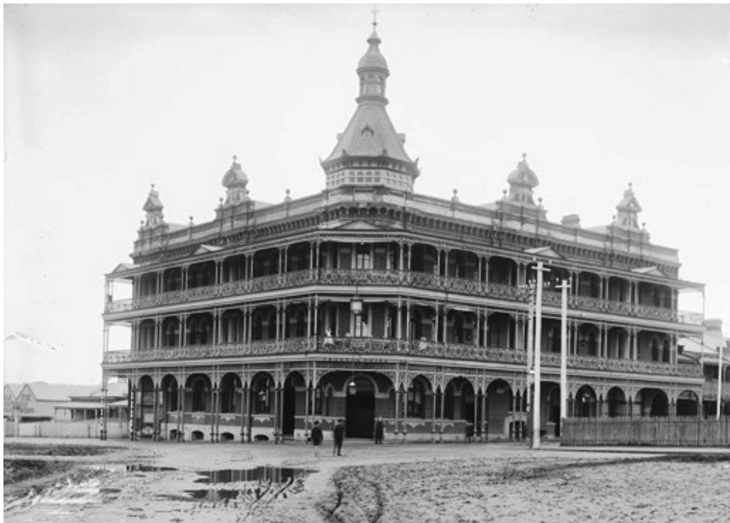
The Federal Hotel on the south-east corner of Wellington and George Streets in Perth, c.1905. Designed for Bernard Stein by James Wright in mid-1896, it was finished in mid-1897. Wright called tenders for 10 villas on behalf of Stein in early 1896, and with this business relationship, may later have been involved in the architectural tuition of Bernard's son, Louis Stein.
