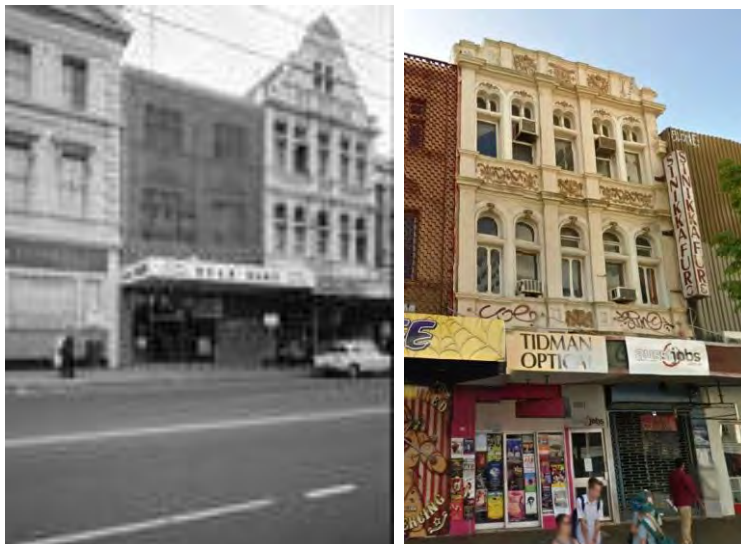
Smith's Chambers at 115-117 Barrack Street of 1897, at right of first photo with gable intact, and in current form with gable removed (SLWA 280017PD, Google 2014)
