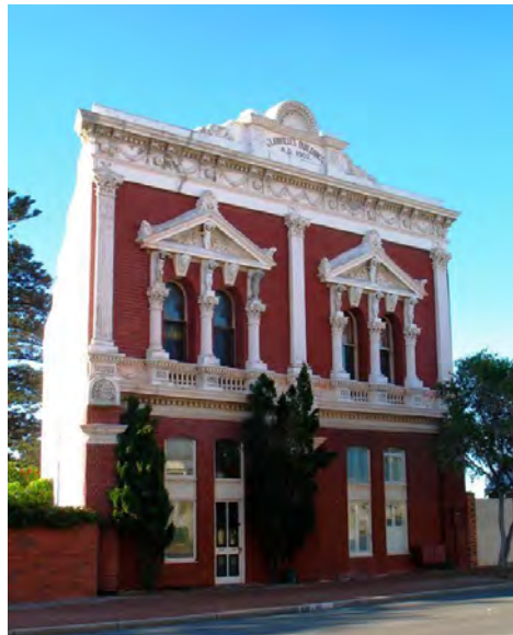
Glanville's Buildings on Canning Highway, East Fremantle (flickr.com, Diana House)
