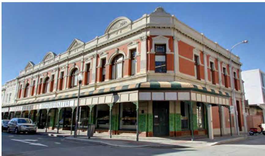
J & W Bateman, later Union Stores, Premises south-east corner High & Henry Streets Fremantle of 1896 (Google 2013)
