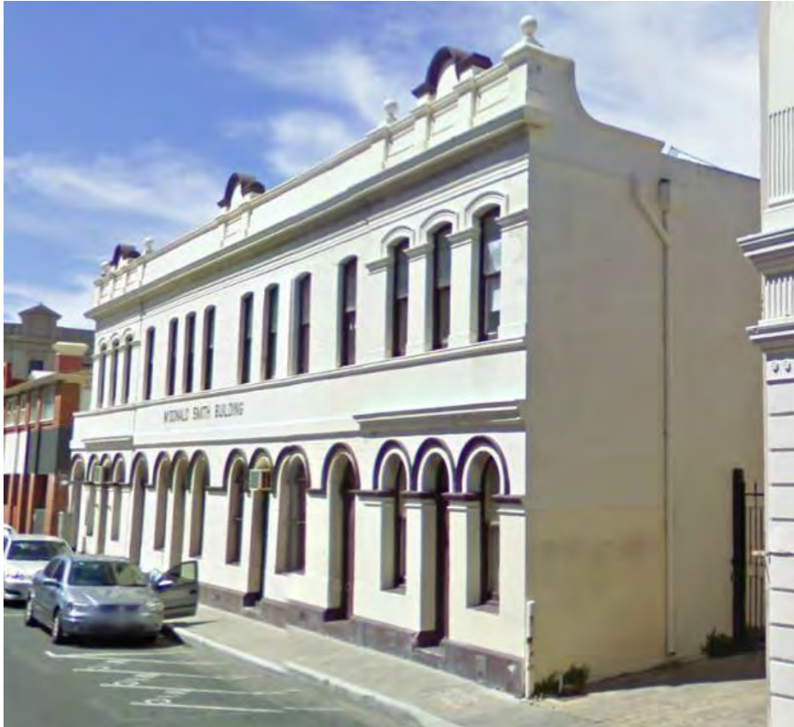
Cliff Street Chambers 22-32 Cliff Street Fremantle of 1896 (Google 2013)
