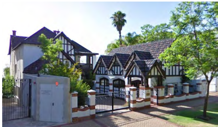
Inter-War Old English style residence at 10 Bellevue Terrace, West Perth credited to H. Bonner [in Molyneux, Ian, Looking Around Perth , RAIWA (WA), 1981, p.56] (Google 2013).
