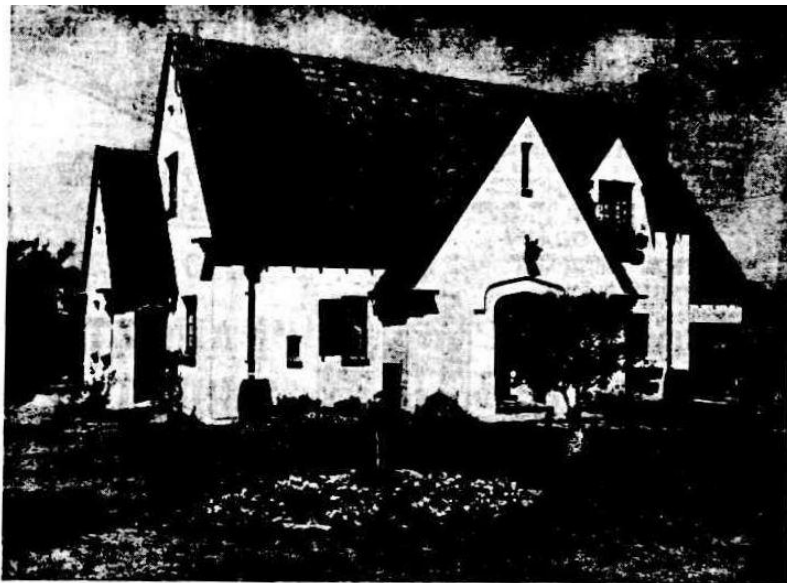
H. Howard Bonner, Esq., Architect.
