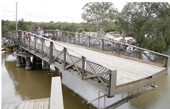
Figure 4. The Restored Sale Swing Bridge
