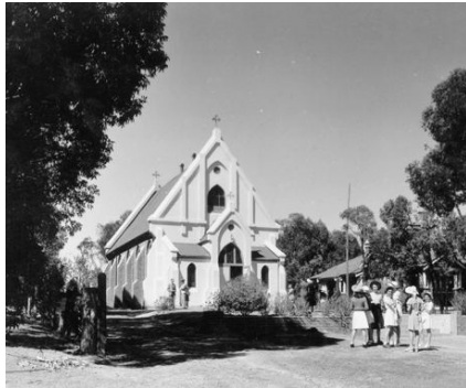
St Matthew's Catholic Church, Narrogin was replaced in 1964 (SLWA 011359D)
