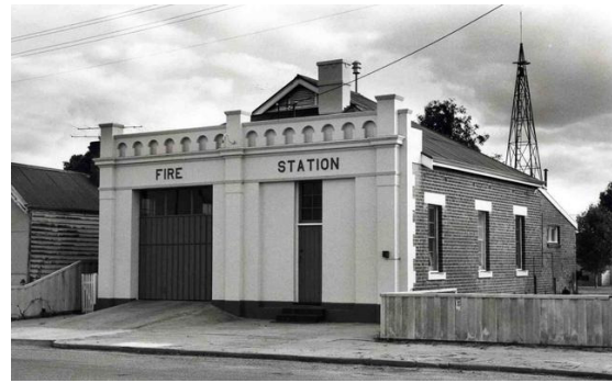
Wagin Fire Station (HCWA Pic4689)
