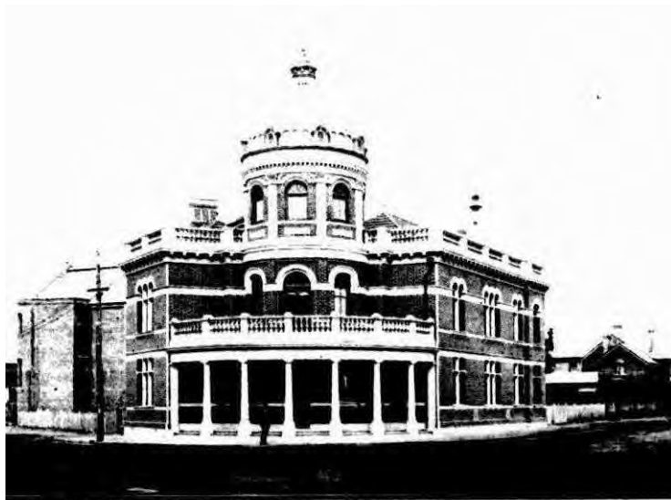
Photo by THE NEW MIDLAND JUNCTION TOWN HALL. OPENED BY THE PREMIER ON JANUARY 23. H. Bodd. Midland Junction.
