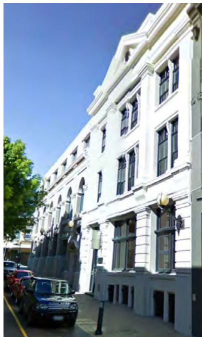
B. Rosenstamm's warehouse 61-65 King Street, Perth 1904 (Google 2013)
