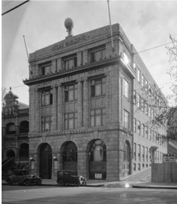
The Atlas Building opened in 1931 at the corner of The Esplanade and Sherwood Court in Perth ( Daily News , 13 March 1930, p.9; SLWA 095428PD)
