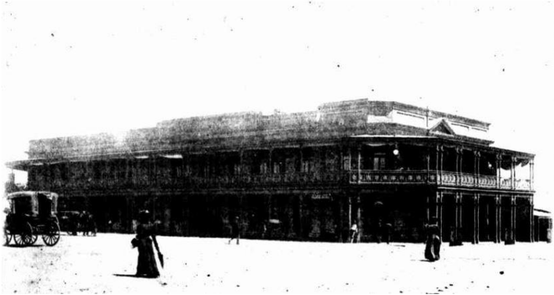
Palace Hotel, Kalgoorlie built in 1897 ( Western Mail , 10 December 1897, p.48).
