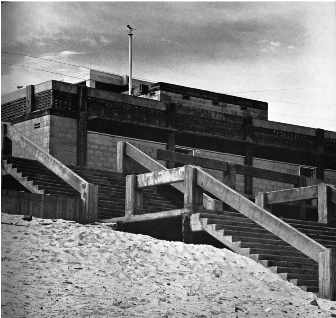
Changing rooms at North Cottesloe Beach ( Towards an Australian Architecture , p.135)
