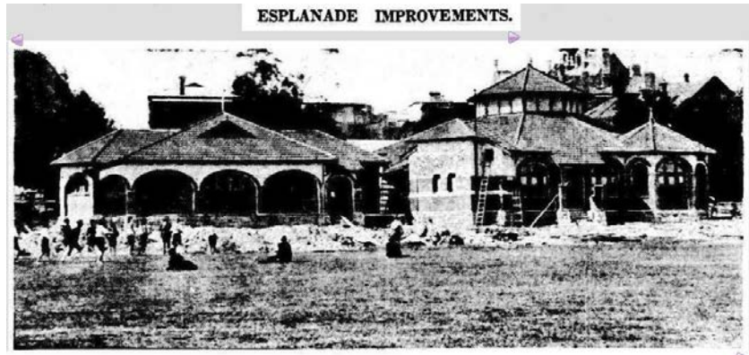
The octagonal refreshment kiosk and dressing rooms (five for men and one for women) facing the Esplanade, close to Barrack-street. The contract price was £5,961. Tenders are being called for the leasing of the premises, which the council is confident will return more than interest on the expenditure, notwithstanding adverse criticism. The architect was Mr. L. B. Cumpston.
