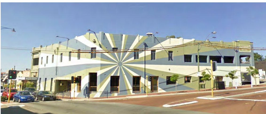
The wrap-around verandahs have been removed and various additions made to the 1902-built Rosemount Hotel, cnr Fitzgerald and Angove Streets North Perth (Google 2013).
