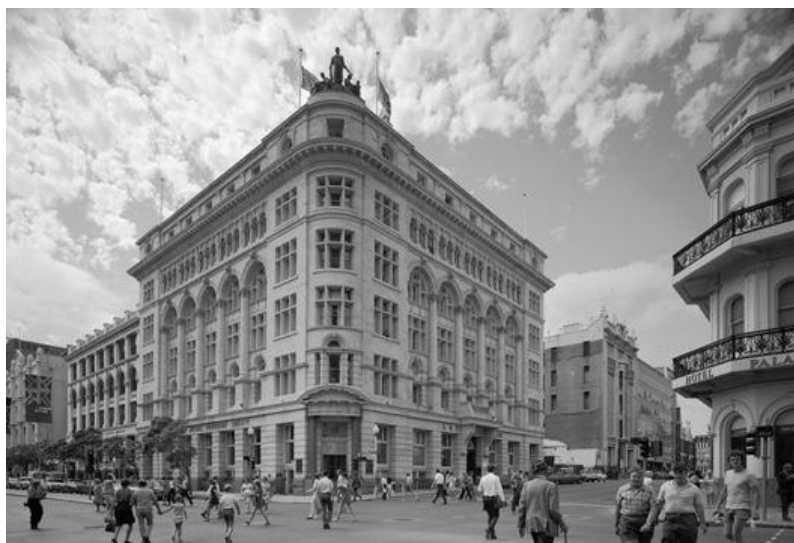
AMP Building, cnr St George's Terrace & William Street, Perth, shortly before its demolition in 1972 (Fritz Kos SLWA 341133PD)
