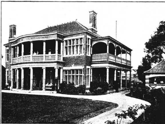
Lexbourne House, Colin Street, West Perth ( The Salon , July 1915, p.210)
