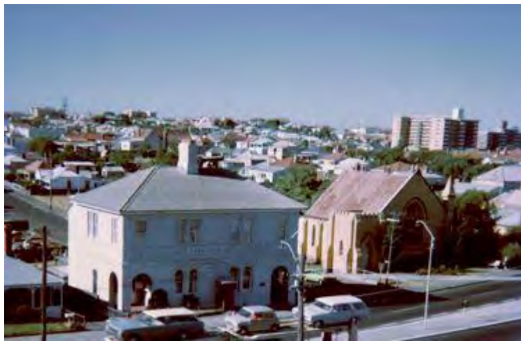
The tower Burwell illustrated in the Western Mail during 1899 for the Presbyterian Church at East Fremantle was never completed. The church is shown in the photo above, to the right of the former East Fremantle Post Office, but it has since been demolished (SLWA 133970PD).
