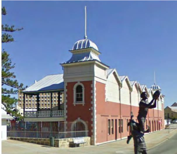
Fremantle Oval Grandstand, Parry Street Fremantle 1897 (Google 2013)
