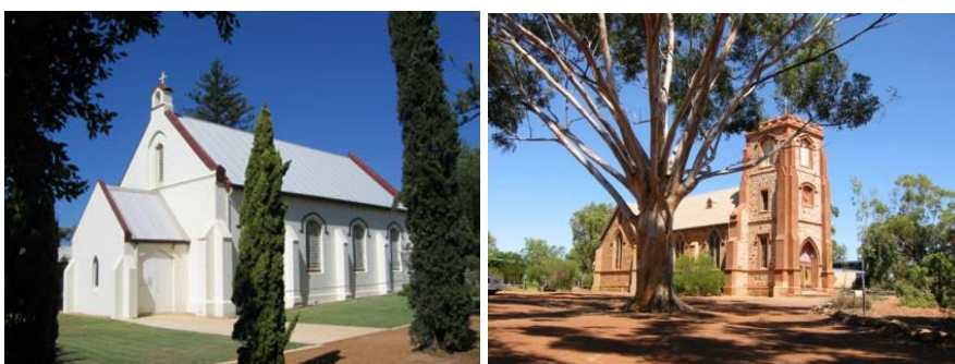
St John the Baptist Church, Dongara (John Taylor); St John's Church, Northam (HCWA)
