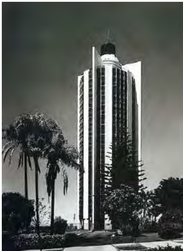
Mount Eliza Apartments of 1964, West Perth effectively marked the change in generation from Harold Krantz to son David ( http://watvhistory.com/2012/06/remembering-dorothy-krantz/ ).
