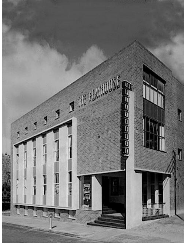
The Playhouse Theatre, Pier Street Perth opened in 1956, and was demolished in 2012 ( http://watvhistory.com/2012/06/remembering-dorothy-krantz/ )
