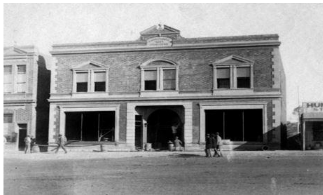
Coolgardie Chambers, Bayley Street Coolgardie under construction in 1895 (SLWA 009092D)
