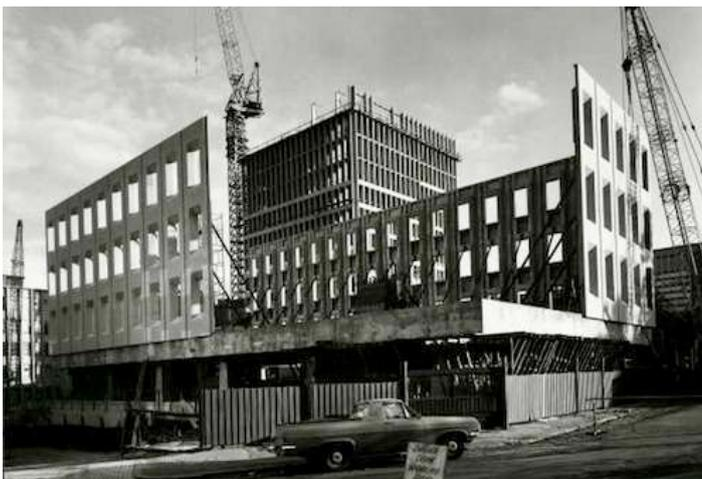
Placing pre-cast panels to rear building, 1967, by Wolfgang Sievers [SLV]
