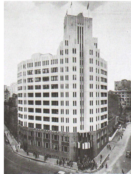
Bligh and Hunter Street facades (Source: Building , October 1936, p. 28)
