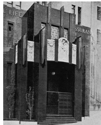
Main Entrance (Source: Building , October 1936, p.30)
